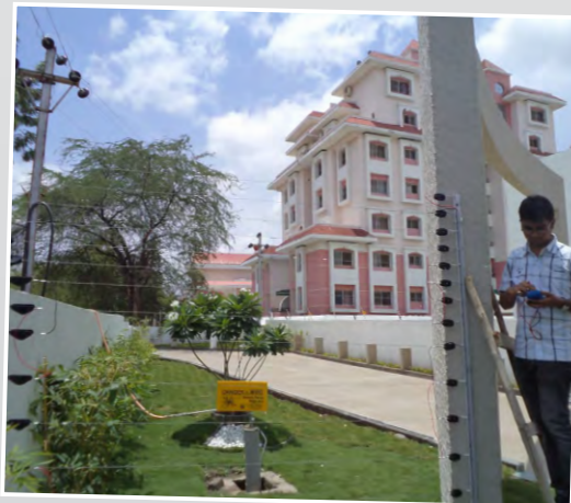
Security Fence Installation, India
